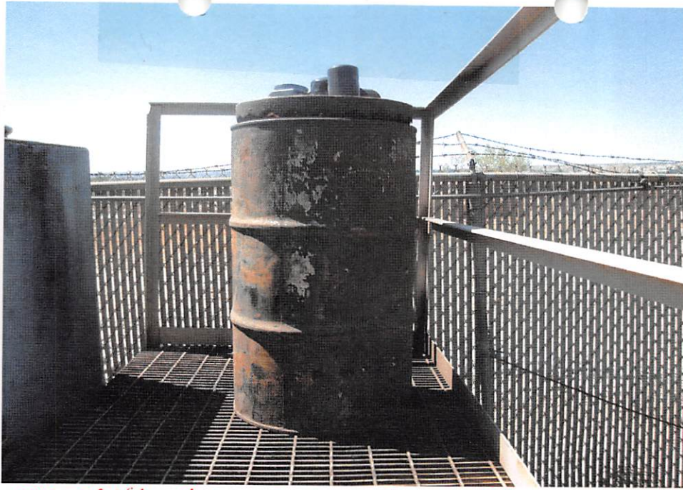
279.22(Cc)(i) - Failure to label "used oil"
