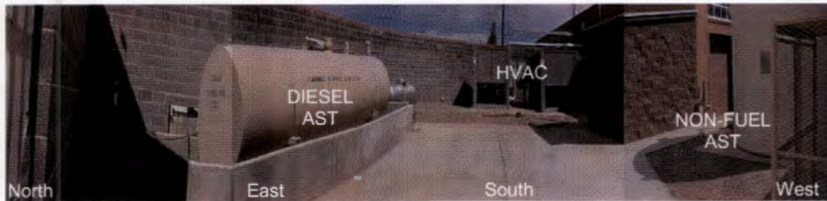
Photograph 2. Inside View of Hospital AST Area
