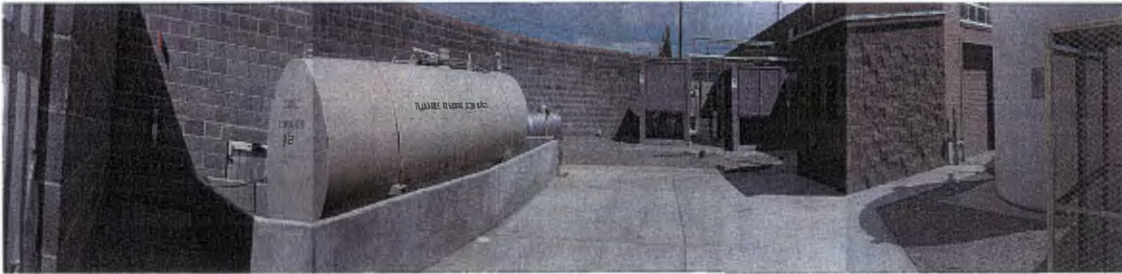
Photograph 2. Inside View of Hospital Area
