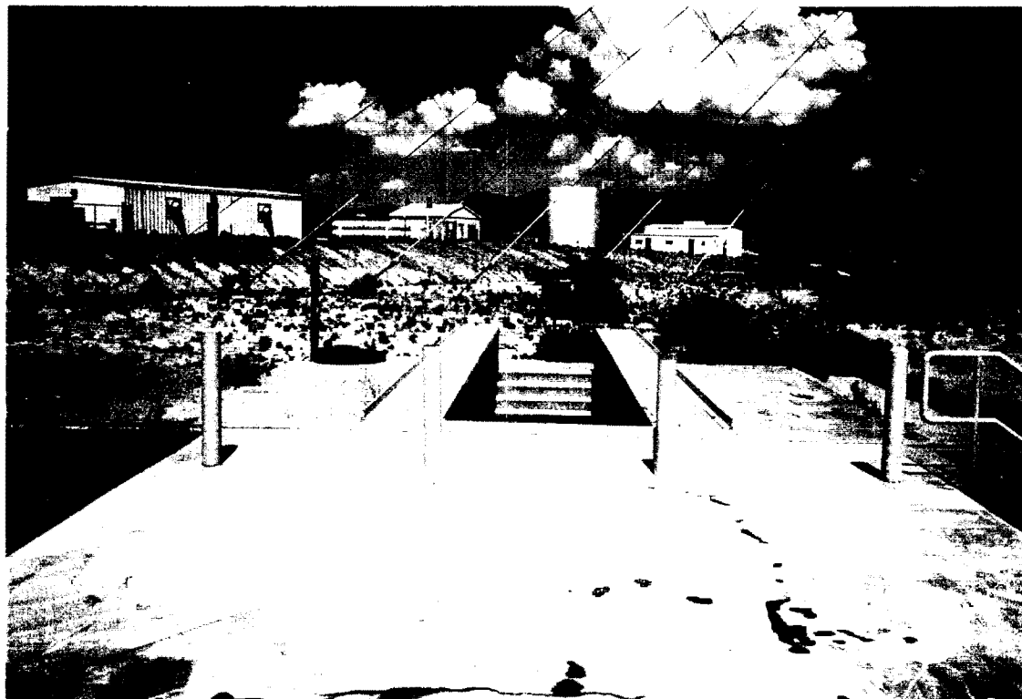
Figures 3-4. Photo Showing Vehicle Pit Protective Posts
