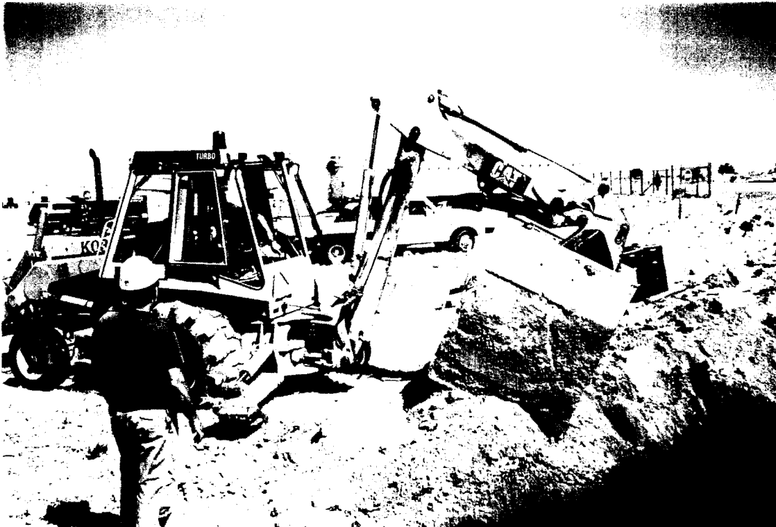
Figure 3-1. Photo Showing OWS Removal
