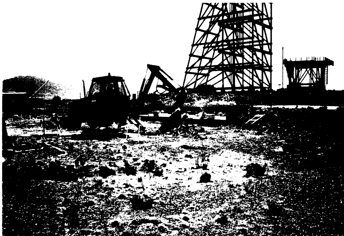
Figure 3-2. Photo Showing OWS Demolition
