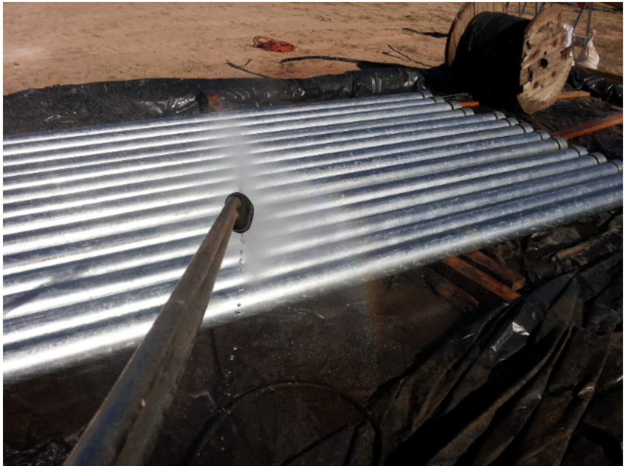
Photo 4. Decontamination of Injection Piping
