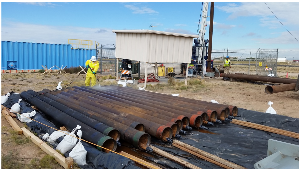
Photo 1. Decontamination of KAFB-7 Piping Exterior
