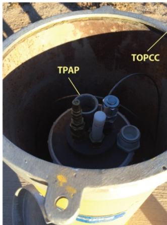
Figure 4. Stick-up well with pump assembly
