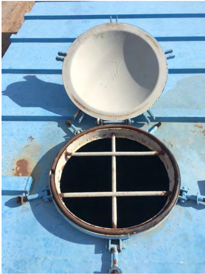
Photograph 1 – Storage Tank Port That Overflowed
