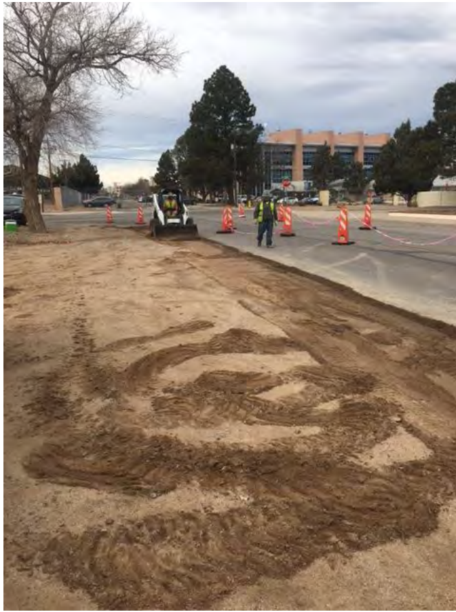
Photograph 5 – Soil Removal Activities – One-Inch Layer, January 9, 2017
