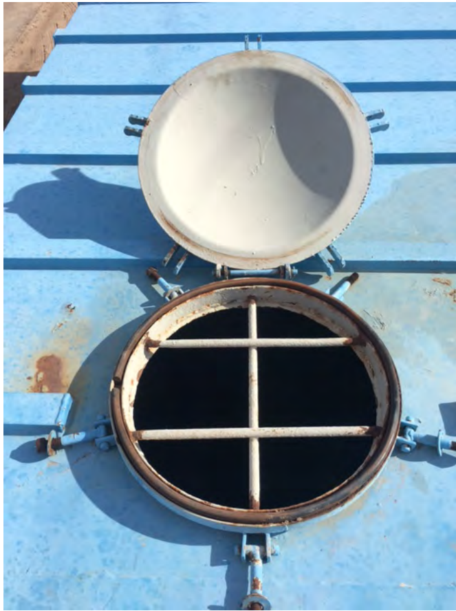
Photograph 1 – Storage Tank Port that Overflowed
