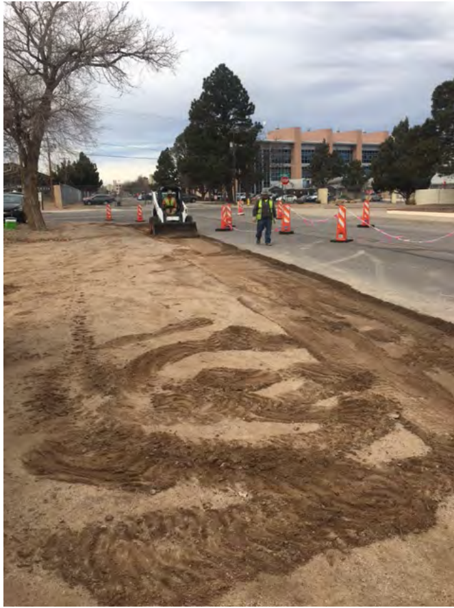
Photograph 5 – Soil Removal Activities – 1-Inch Layer, 9 January 2017
