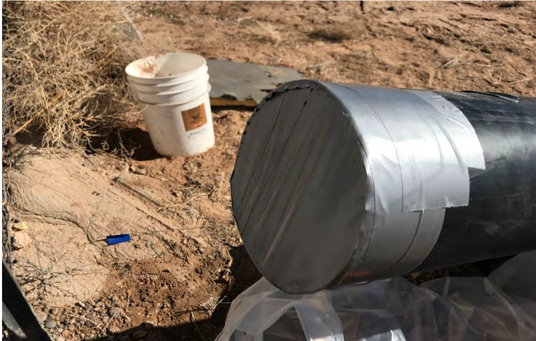
Address: BFF Kirtland AFB Description: Overnight cover for exposed pipe section. Date: February 1, 2017
