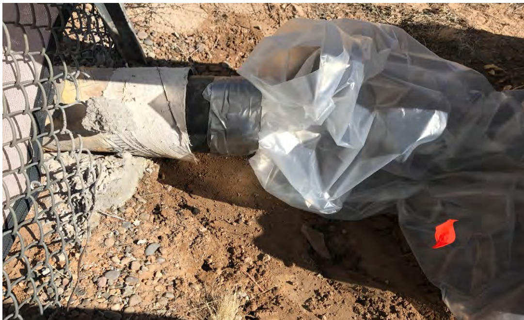
Address: BFF Kirtland AFB Description: Overnight cover for exposed pipe section. Date: February 1, 2017
