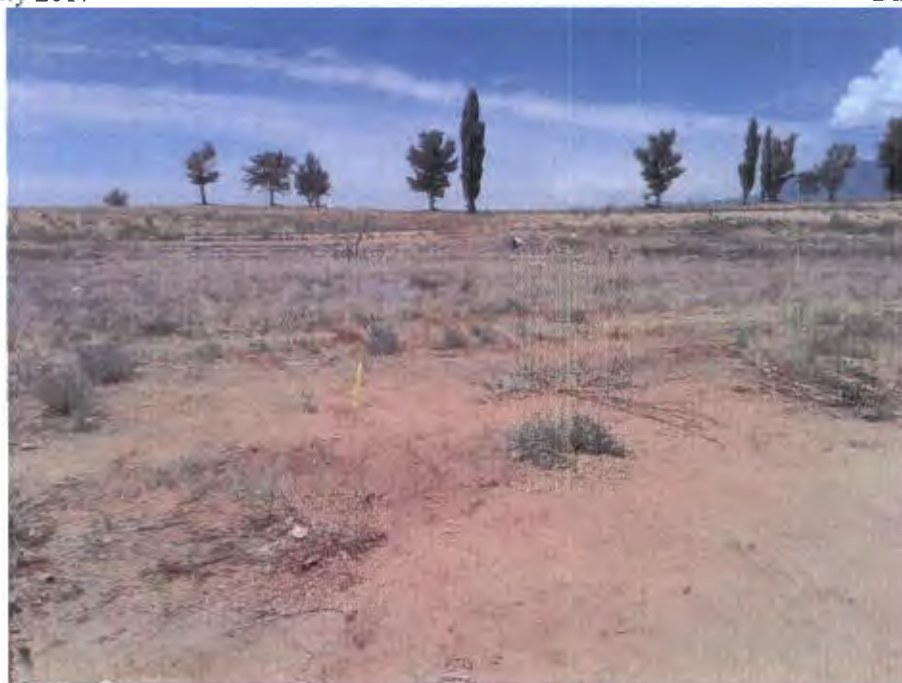
Location: Location 2 Description: Location 2 Post Soil Removal Date: 12 July 2017
