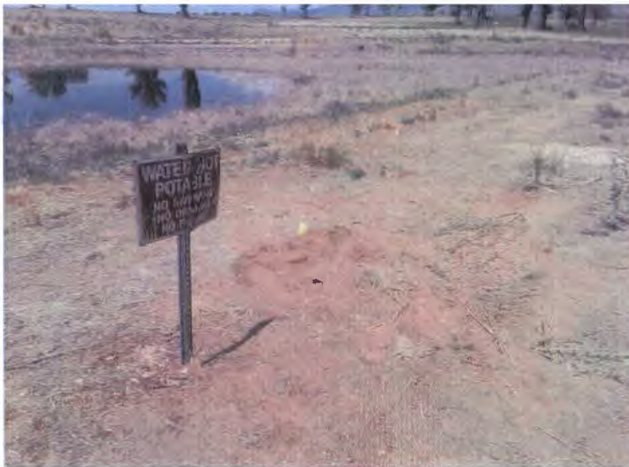
Location: Location 1 Description: Location 1 Post Soil Removal Date: 12 July 2017
