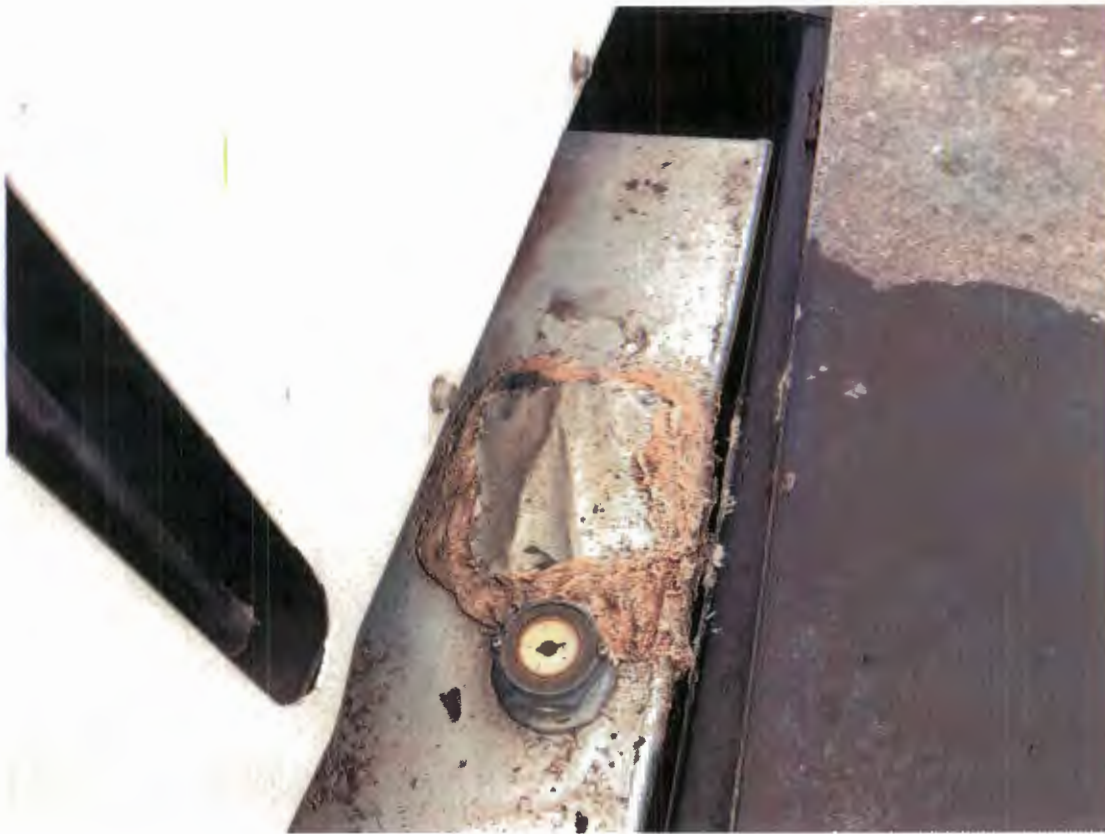
Silicone patch on topside of lower fuel tank
