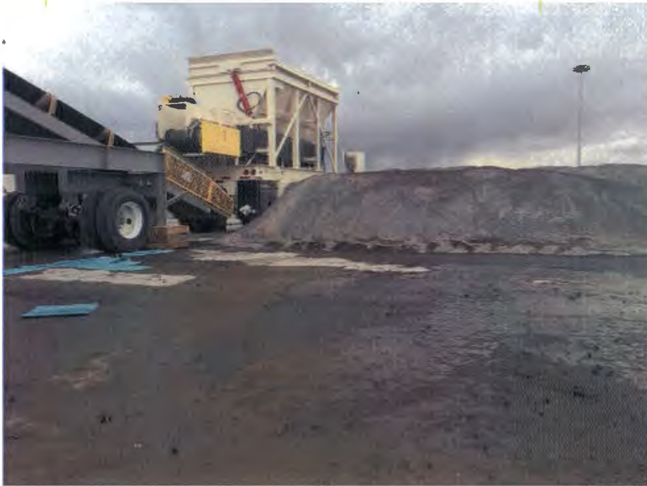
Spill looking east from generator
