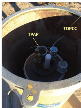
Figure 4. Stick-up well with pump assembly
