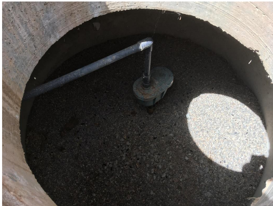
Location: Along Effluent Conveyance Line (Photograph 4 on Figure 1) Description: Air Relief Valve Date: April 04, 2018
