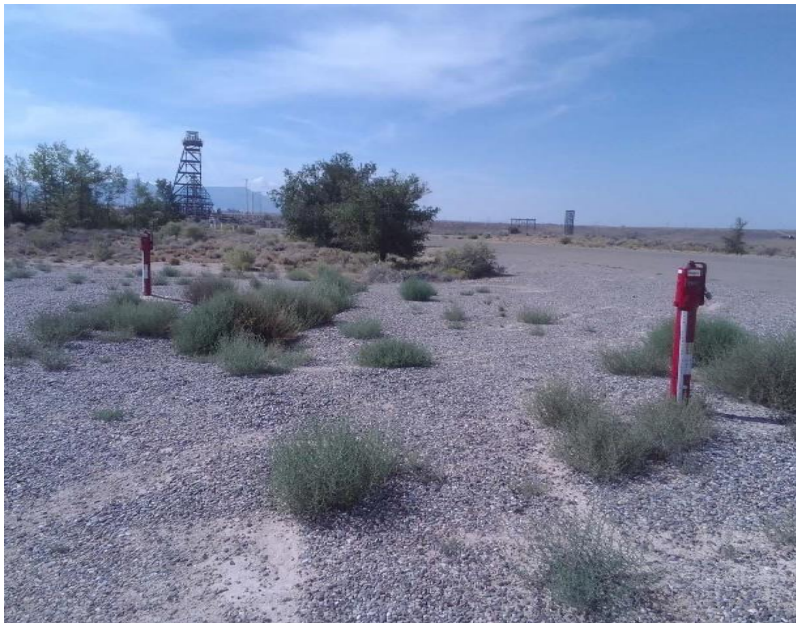
Location: Changeover Valves (Photograph 2 on Figure 1) Description: Post Indicators for the Changeover Valves Date: April 04, 2018
