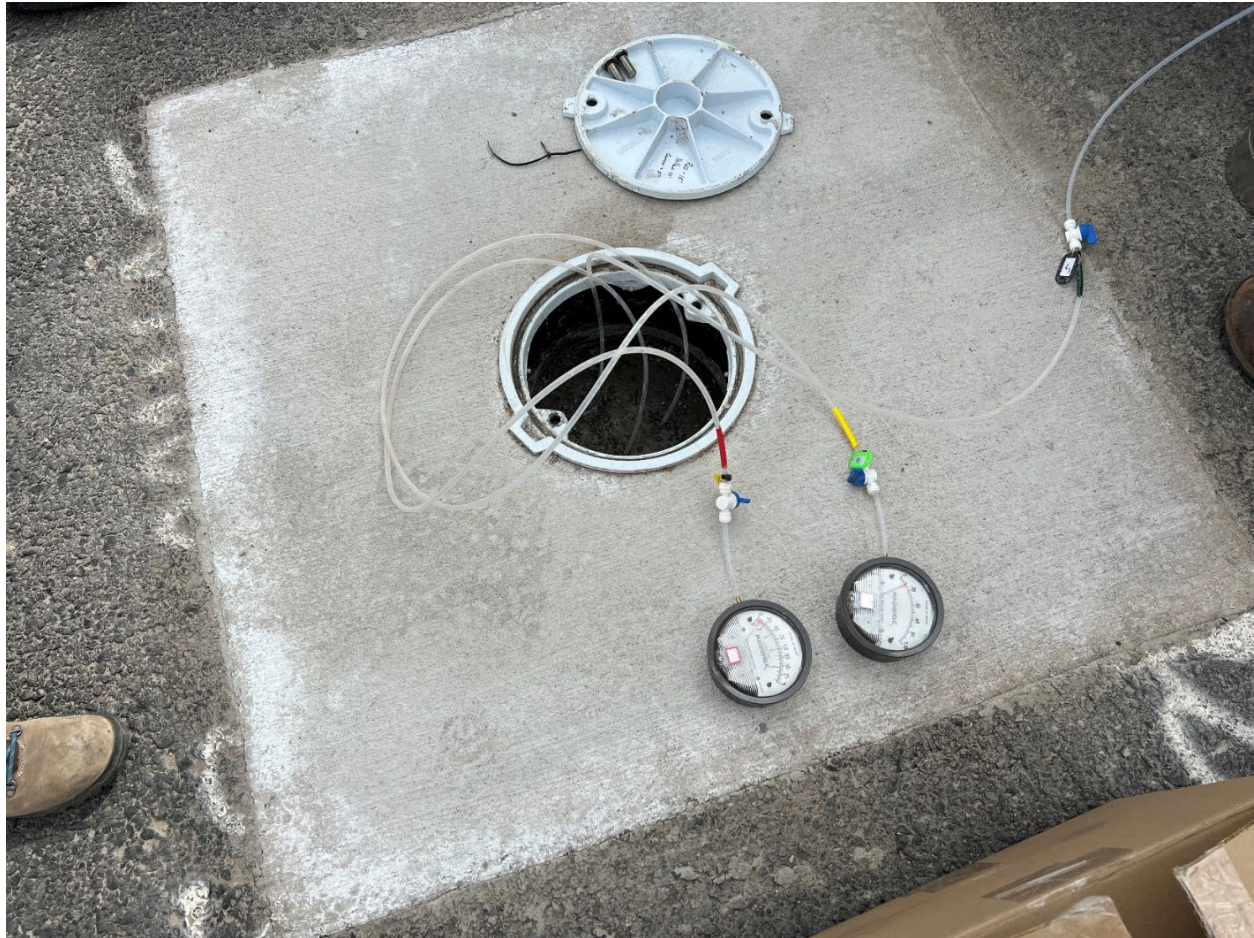
Figure 5-7: Well Vault and Concrete Surface Slab Placement Photo
