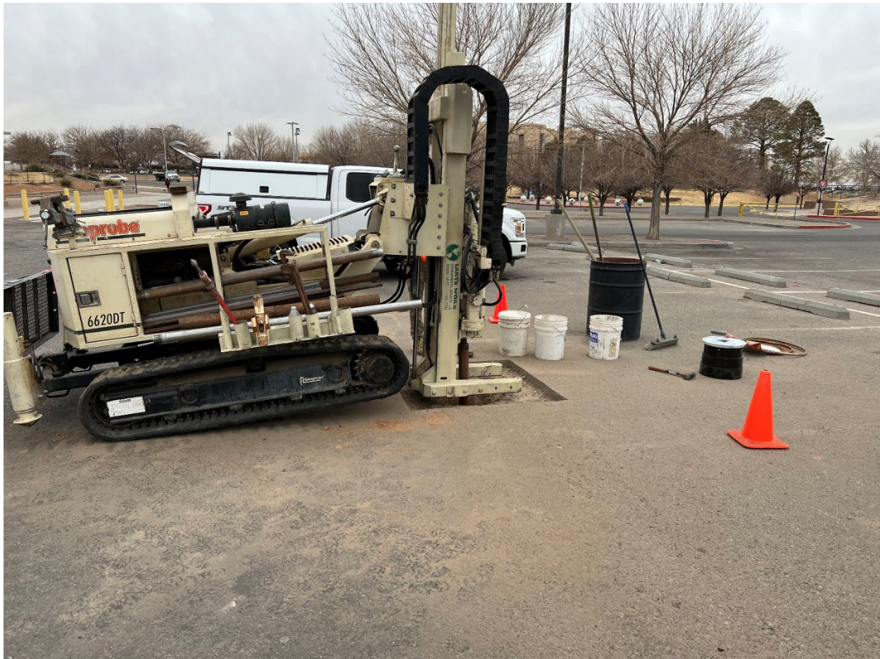
Figure 5-4: Drill Rig Photo
