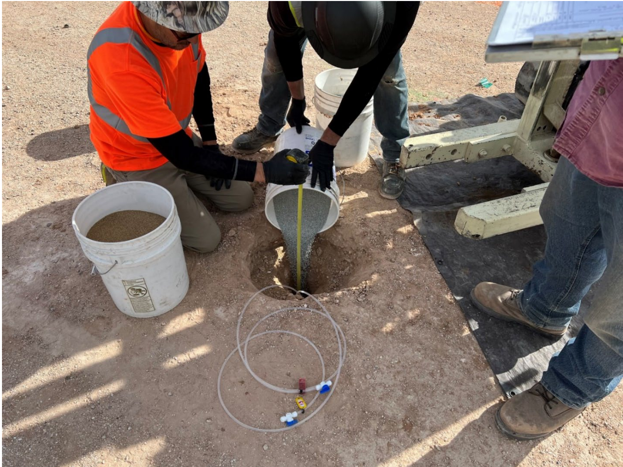
Figure 5-5: Annular Seal Placement Photo
