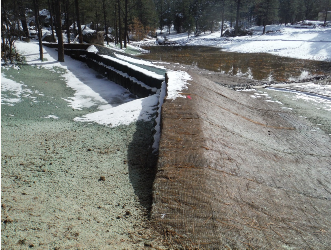
Sandia wetland run-on control and grade-control structure looking southeast, December 5, 2013
