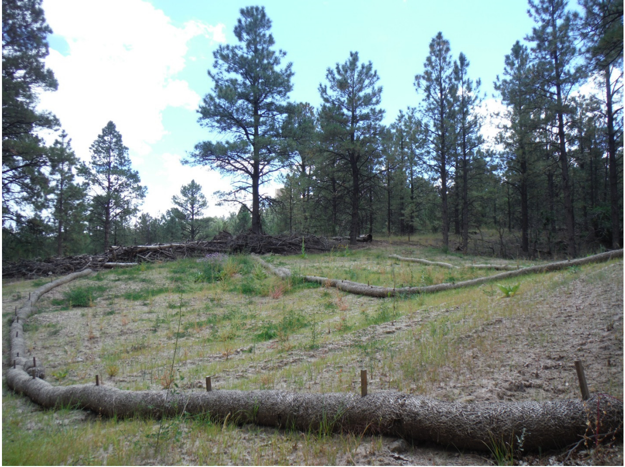
Erosion controls at south-entering swale looking southeast with established vegetation and no signs of erosion or rilling taking place, September 23, 2014
