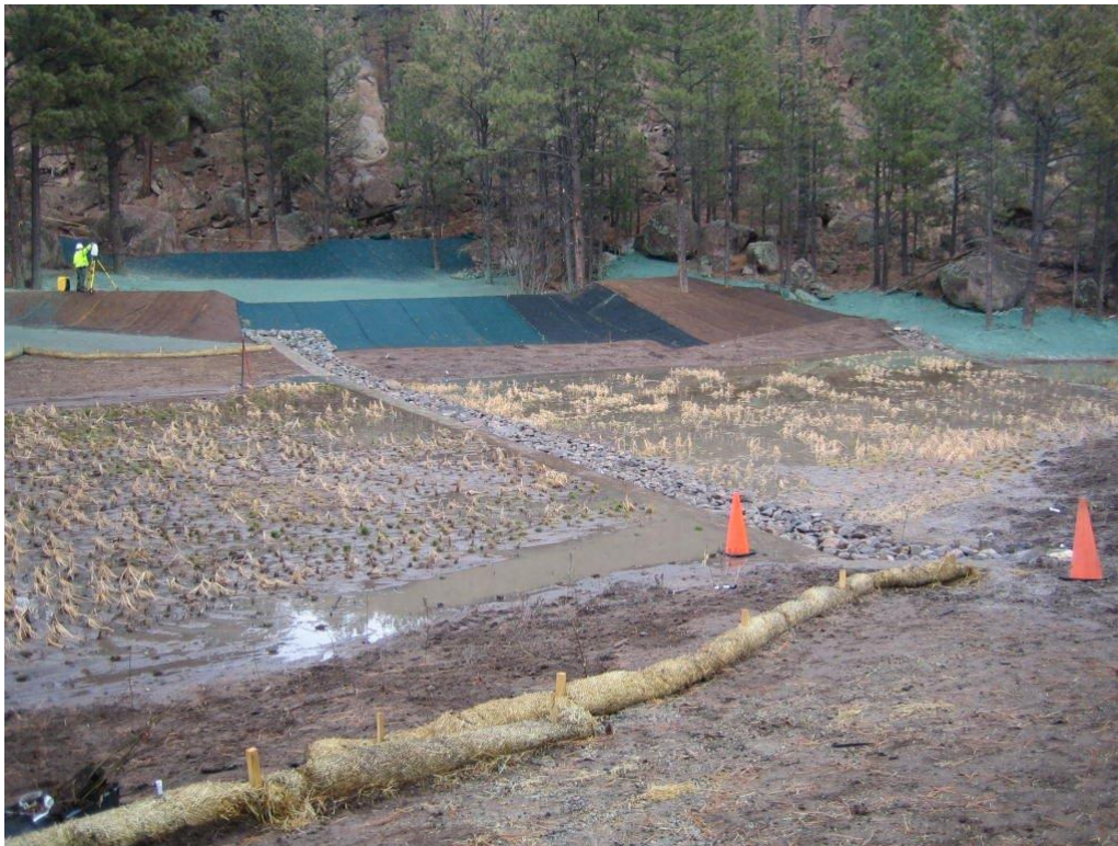
Sandia wetland run-on control and grade-control structure looking north, November 21, 2013
