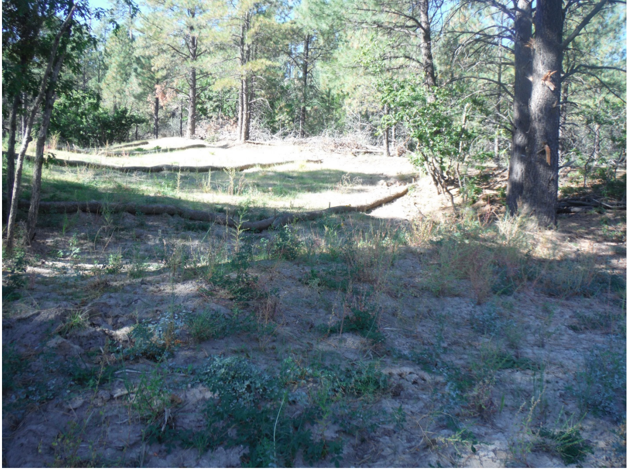
Earthen berm erosion control below south-entering swale looking south with established vegetation and no signs of erosion or rilling taking place, September 23, 2014
