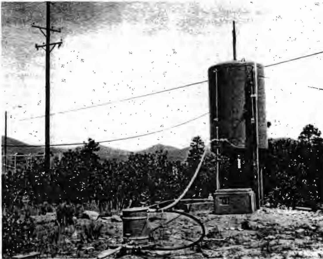
Fig. 6. Storage tank and constant head device.
