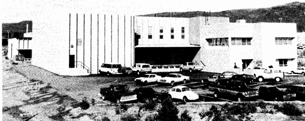
Los Alamos Treatment Development Facility, which houses the controlled-air incinerator.
