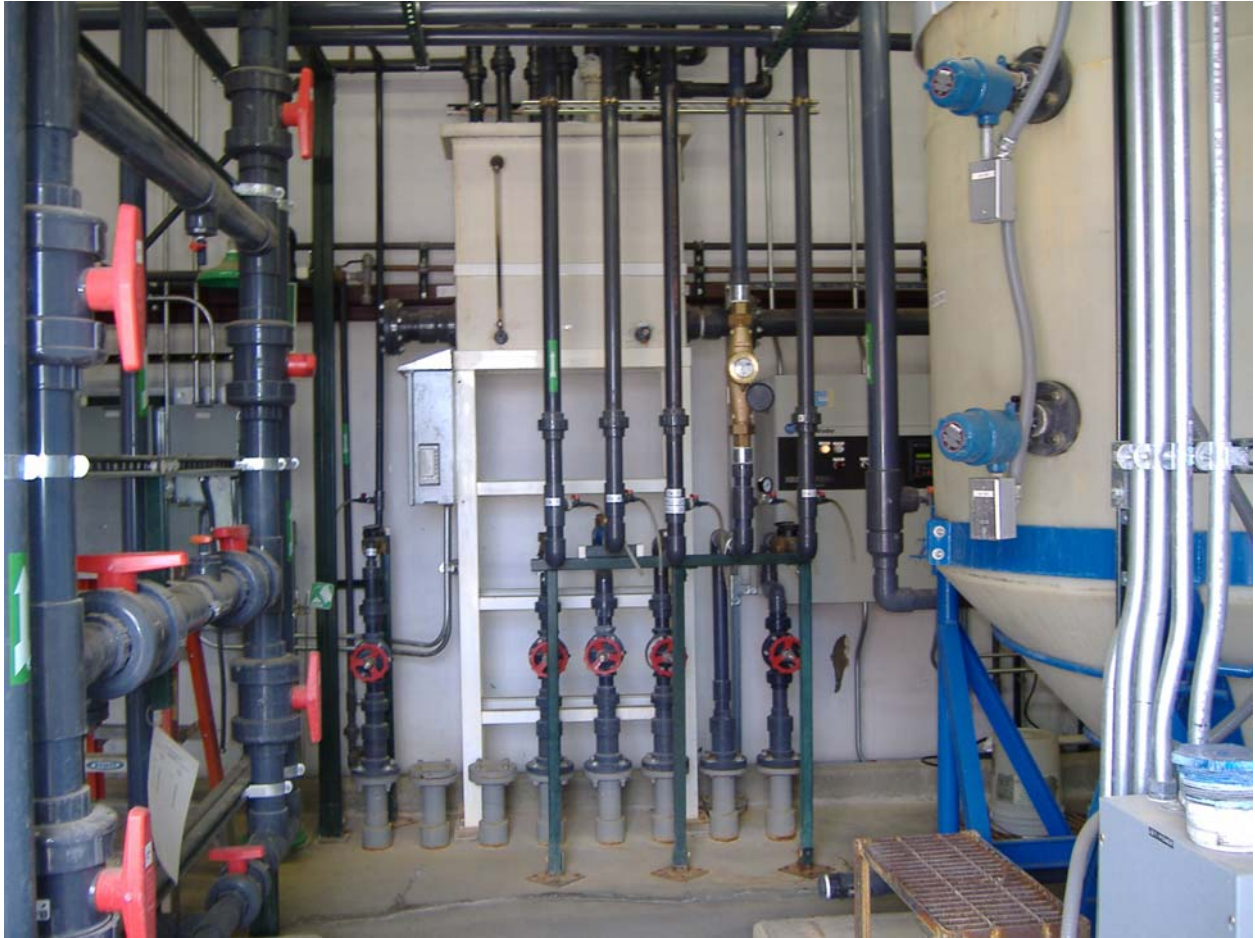
Photo 2 Groundwater Treatment System, Influent Pipes Person Generating Station
