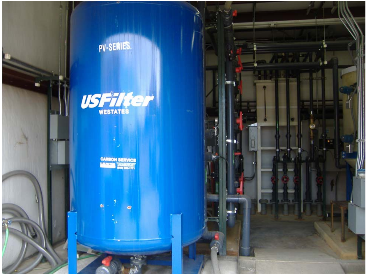
Photo 1 Groundwater Treatment System, Carbon Unit Person Generating Station
