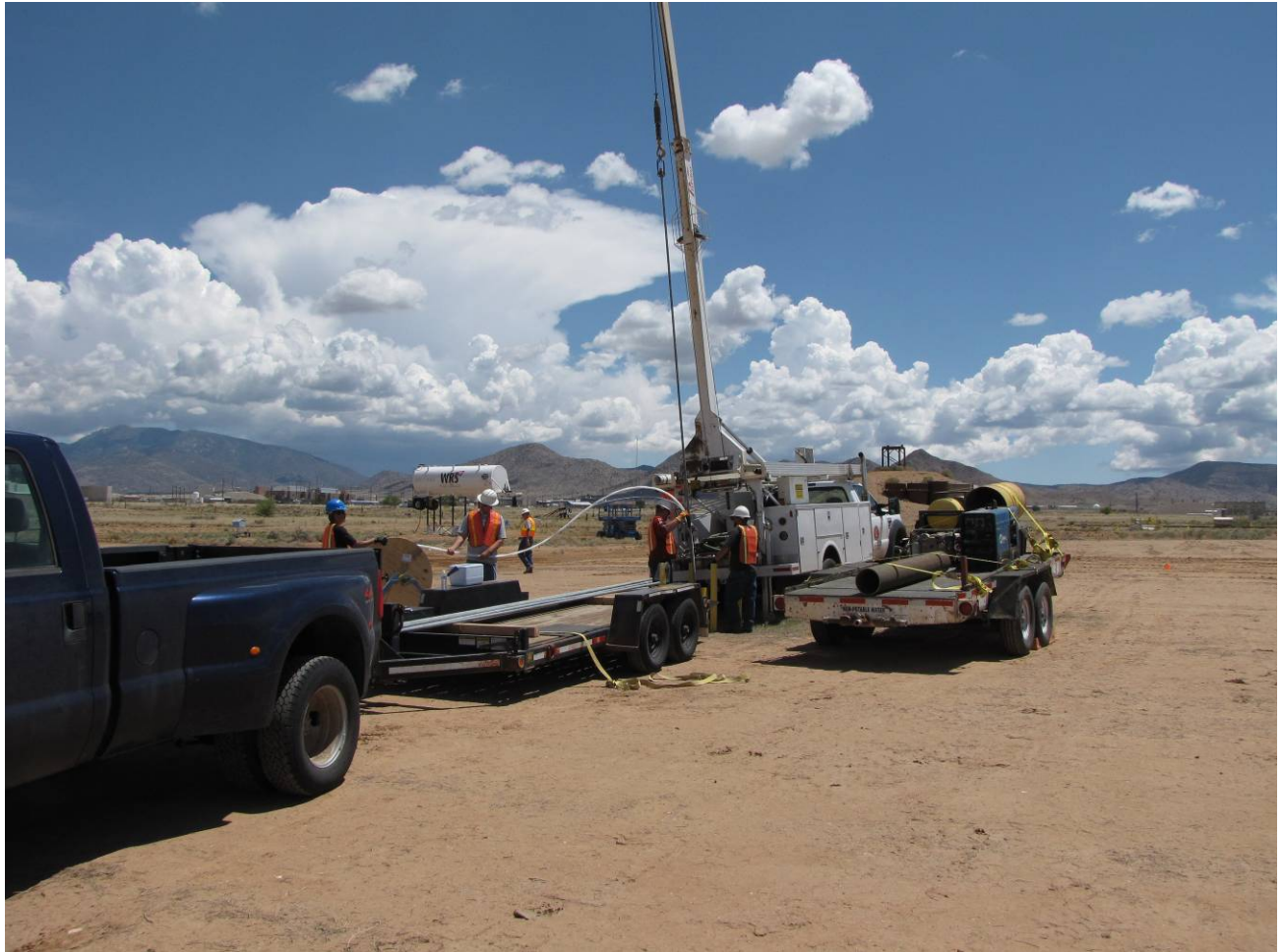
Figure 2-1 Removing the packer assembly from well MWL-MW4, May 27, 2009. View to the east.
