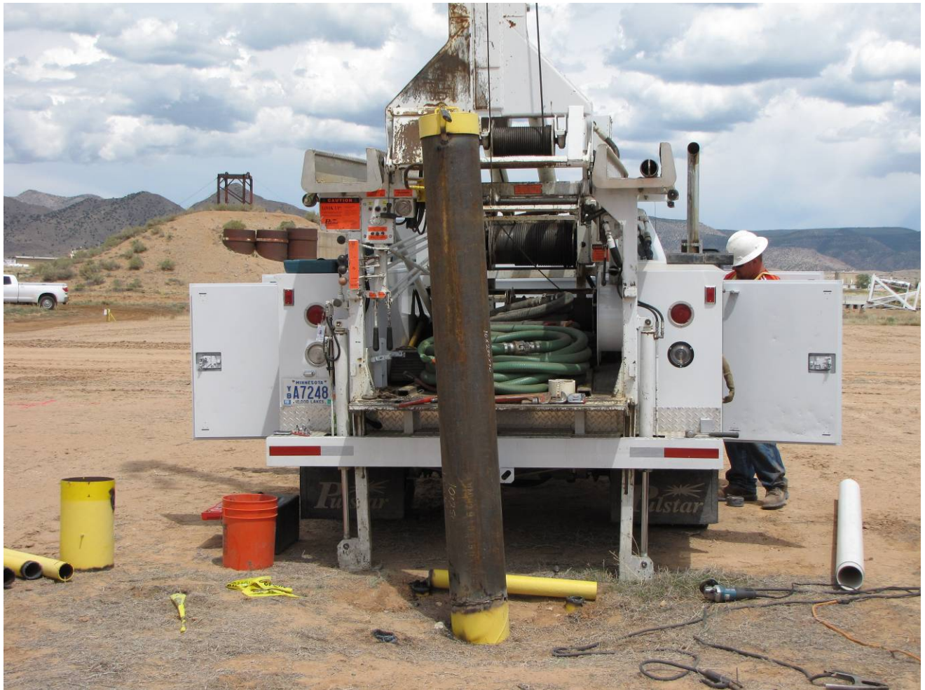
Figure 2-4 MWL-MW4 protective surface casing extension, welded to the existing protective surface casing, May 27, 2009. View to the east.
