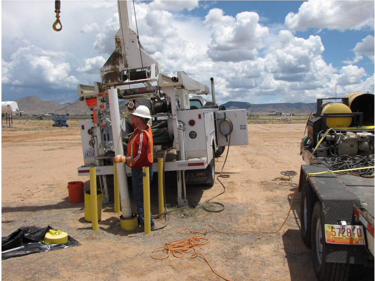
Figure 2-3 Extending the MWL-MW4 PVC well casing, attached to the existing PVC casing with a PVC slip coupling and stainless steel screws, May 27, 2009. View to the east.
