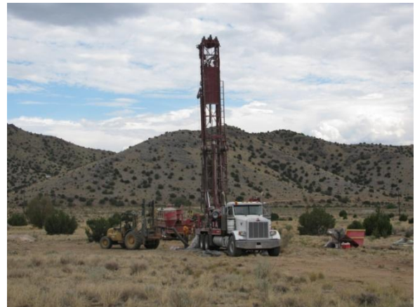
Figure 3 Installation of Monitoring Well CCBA-MW2 at SWMU 58, August 2011
