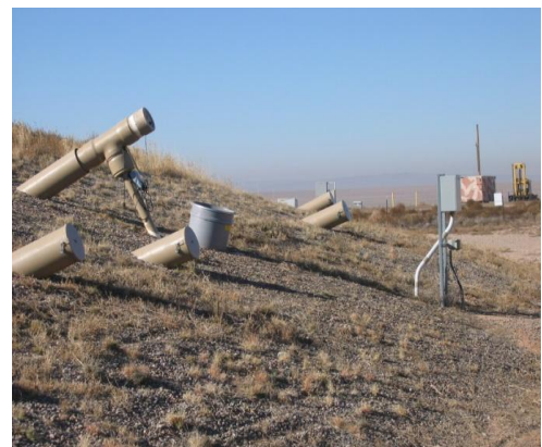
Figure 5 CAMU Leachate Collection and Removal System
