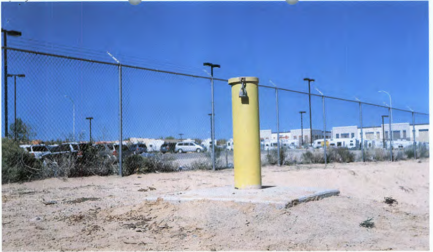
Photo#2 Erosion Repair at MW-72 10-15-2008
