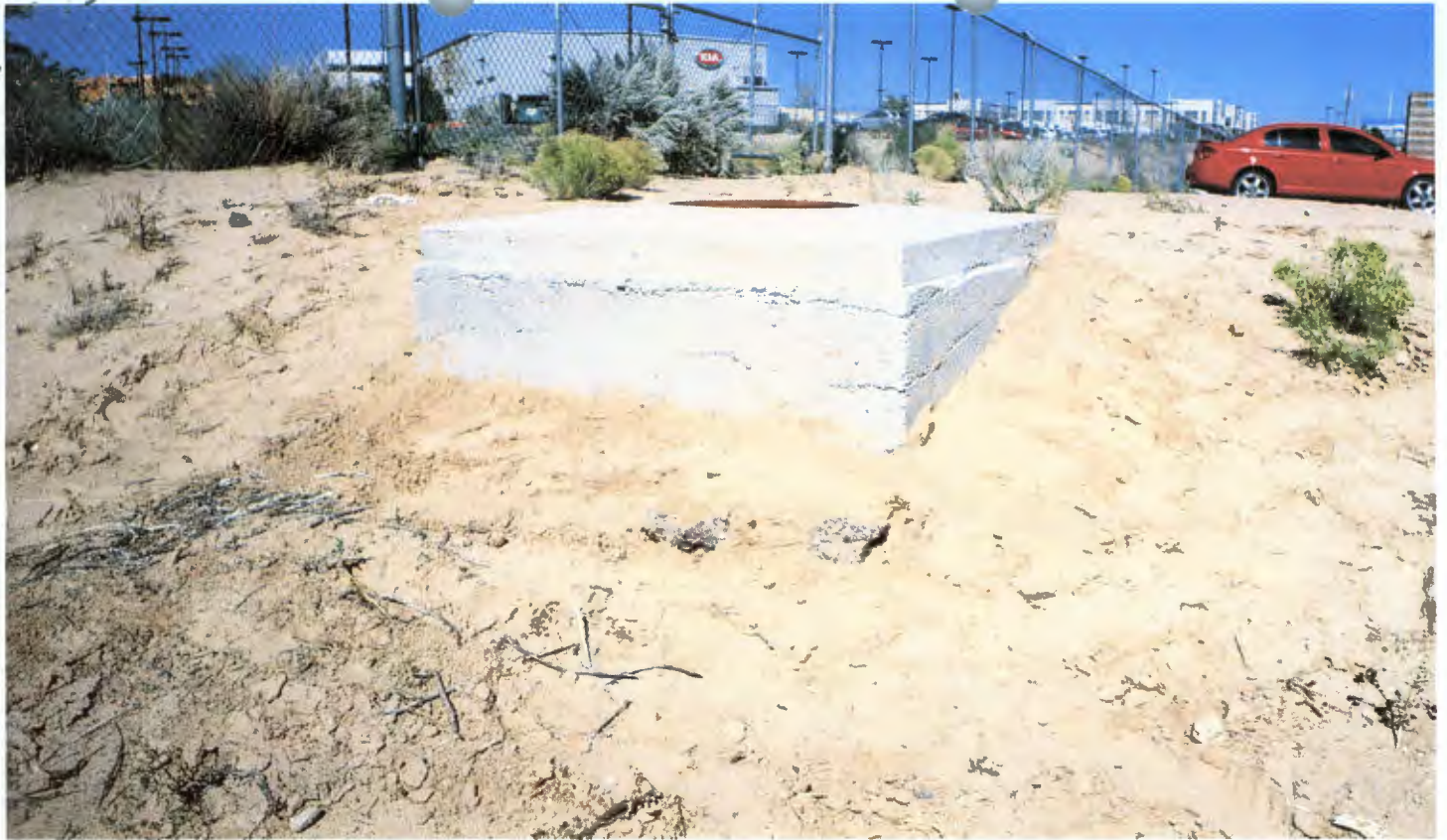
Photo#3 Erosion Repair at MW-73 1015-2008
