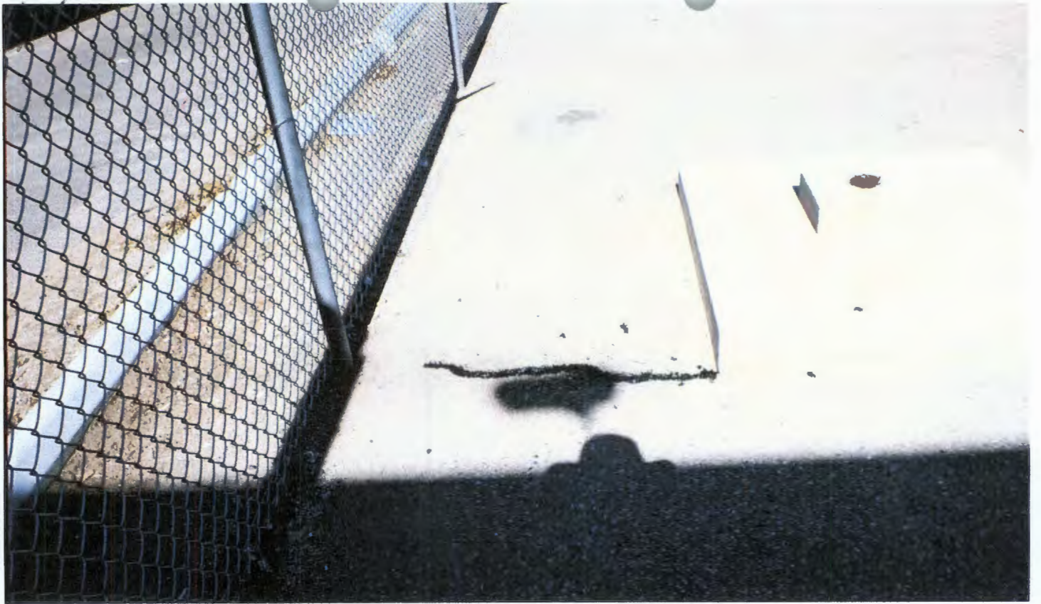
Photo#1 Repaired crack in Capped Ares 10-15-2008
