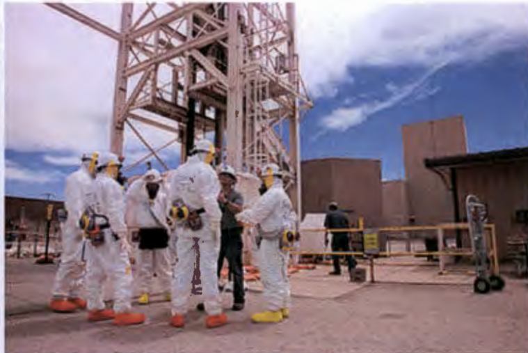
Above: Workers discuss plans prior to entering the underground
