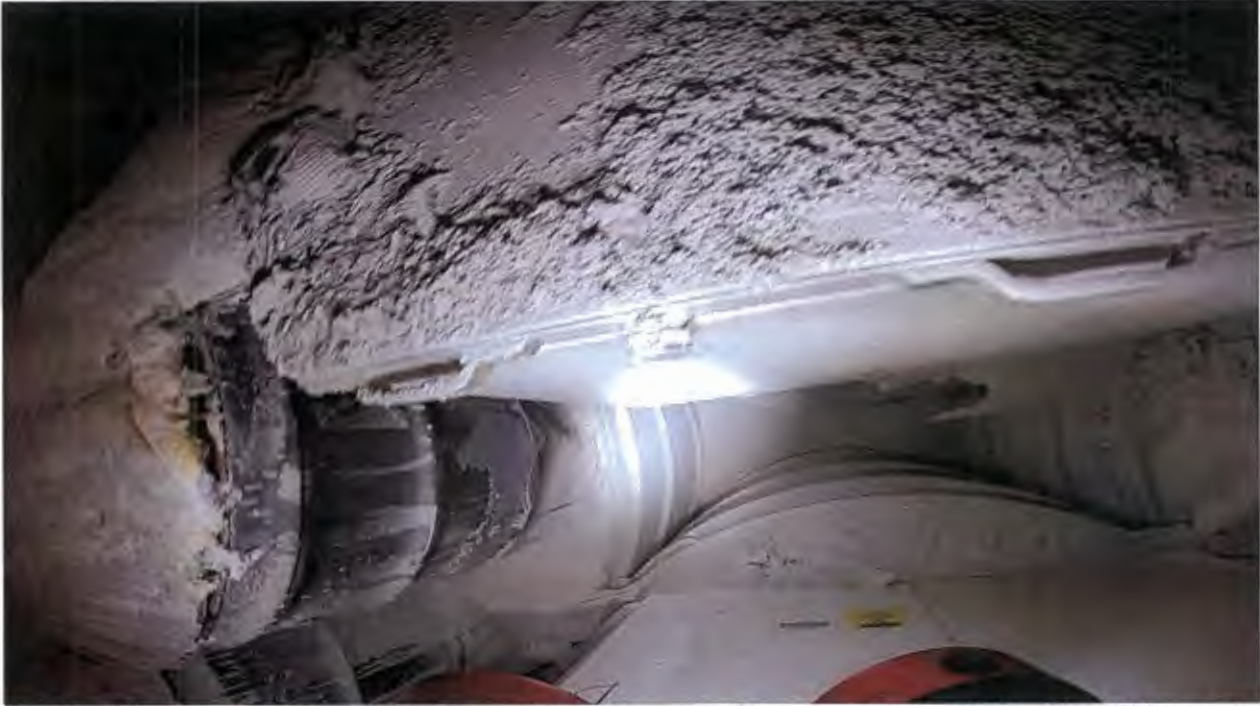
The May 15 entry into Panel 7, Room 7 produced this photo of a waste container (left) with its lid unsealed and apparent heat discoloration.
