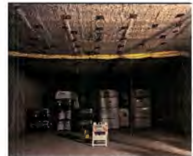
Yellow brattice cloth is suspended from the ceiling in this disposal room. It is rolled down to prevent air flow to the room. Brattice cloth also will serve as a barrier to decontaminate floors.
