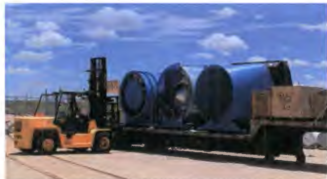
WIPP Employees unload sections of the SVS early this week at the WIPP facility.
