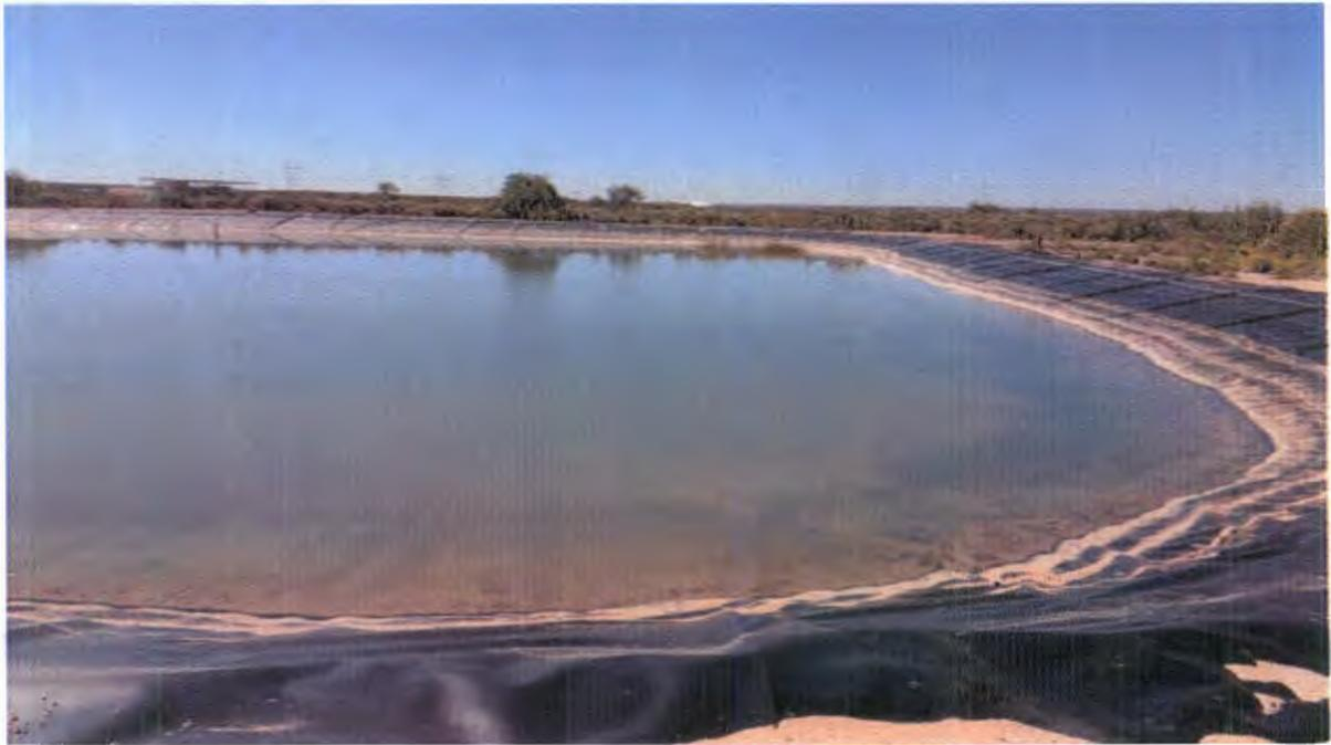
The above and next two pictures show Storm Water Pond 2. WIPP has pumped down Pond 2 and since moved the pump to Storm Water Pond 1. Not the high water marks on the liner.
