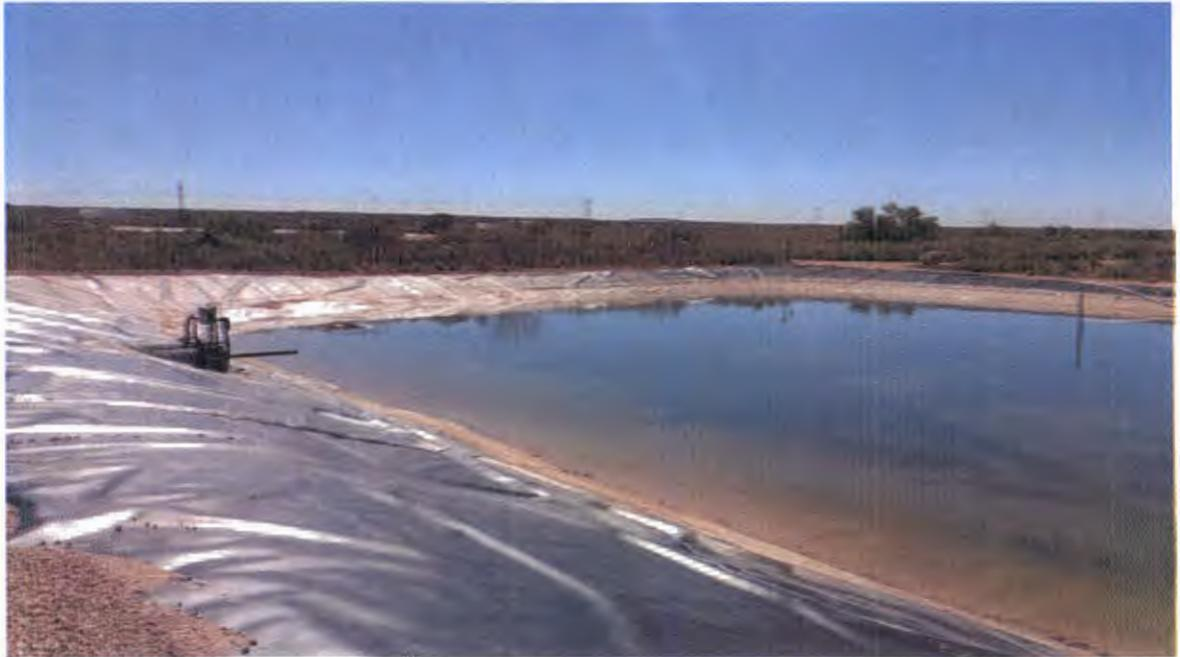
The above picture and following three images show photos of Storm Water Pond 1. WIPP is currently pumping fresh water out of Storm Water Pond 1. Note the high water marks on the liner. Pond 1 did not spill over during the heavy rains, but was very nearly at capacity.
