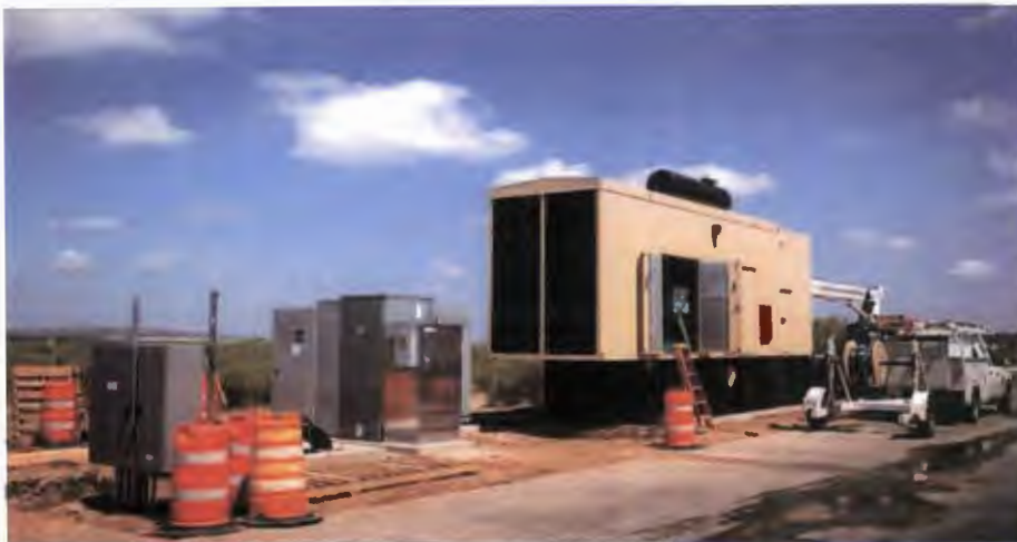
EOC Generator – Under Construction
