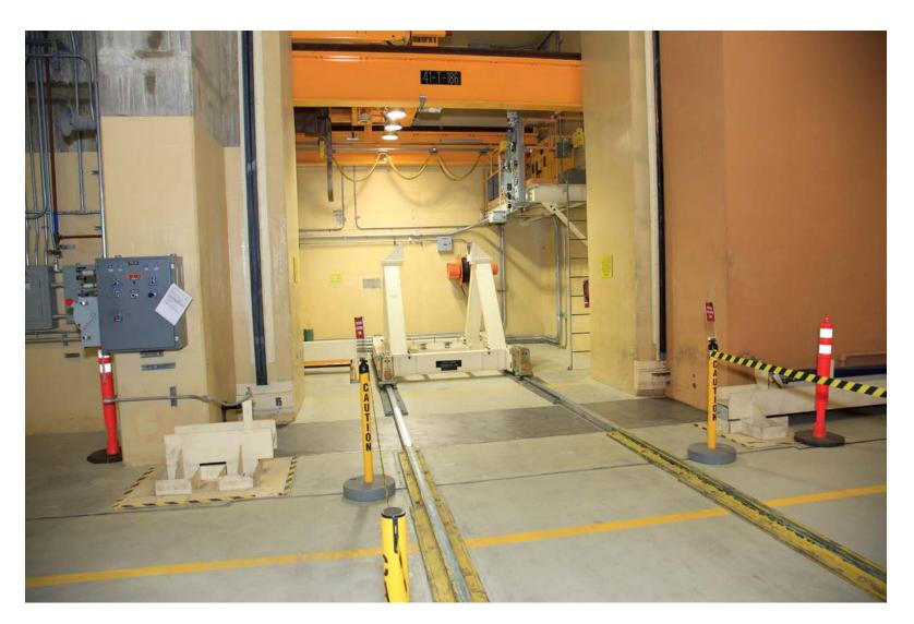
Figure 4-8 Cask Unloading Room and Bridge Crane
