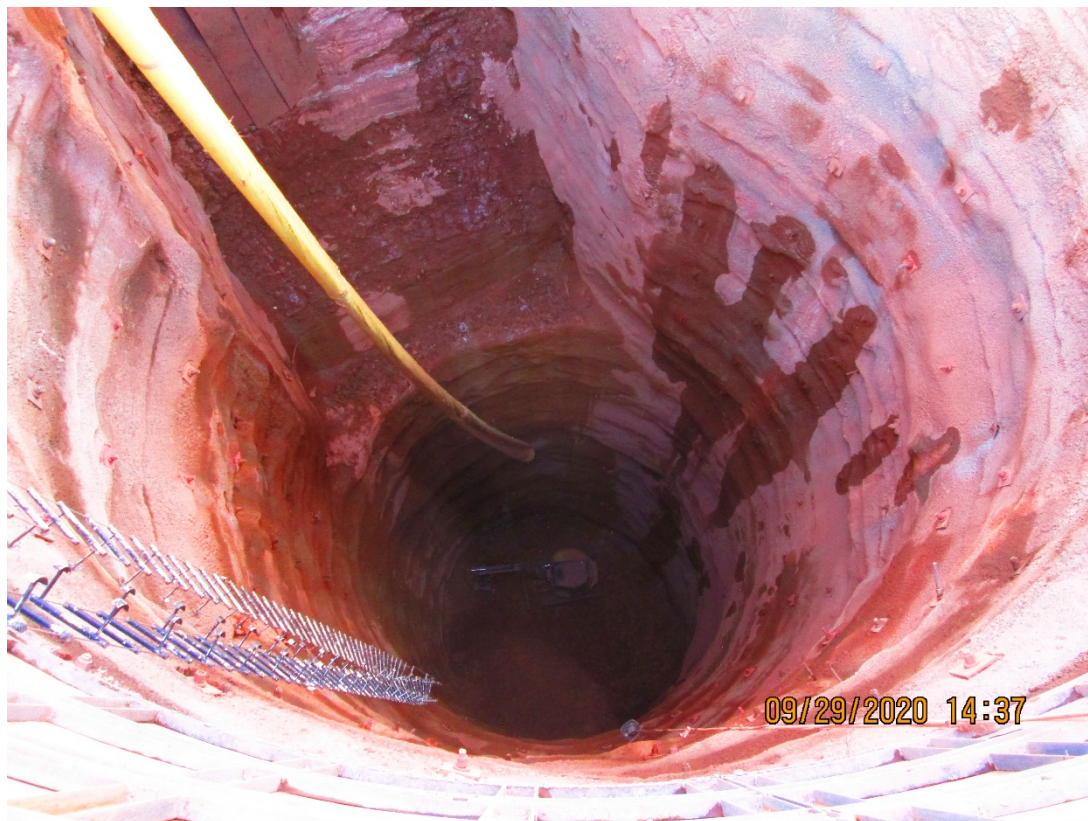
Photo 2: Shaft #5 is 28ft wide and 116ft deep. Notice small backhoe at the bottom.
