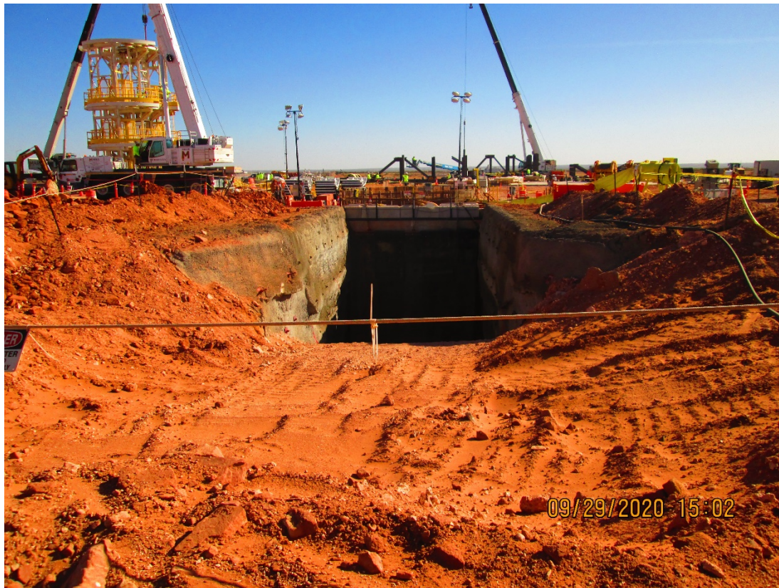
Photo 4: Excavation of plenum area, 45-degree angle that will connect to Shaft #5.
