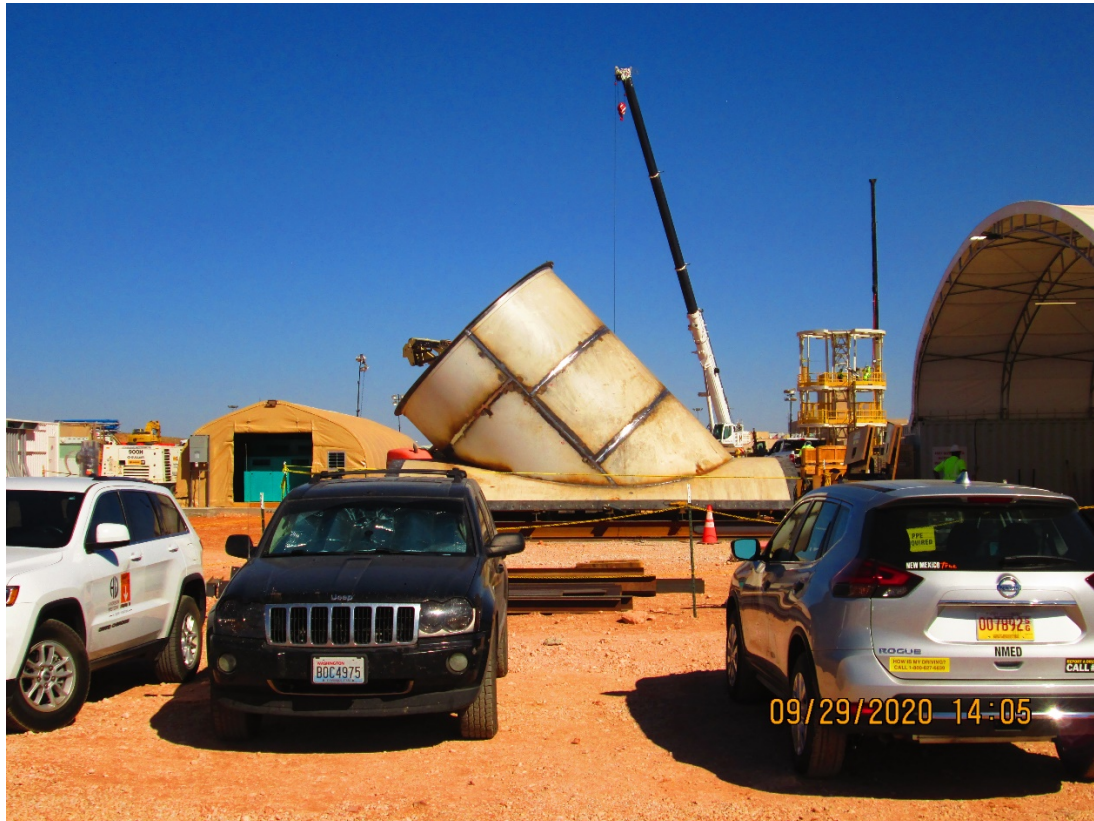
Photo 5: Plenum joint pictured behind vehicles. Plenum joint will connect to Shaft #5 near 50ft depth
