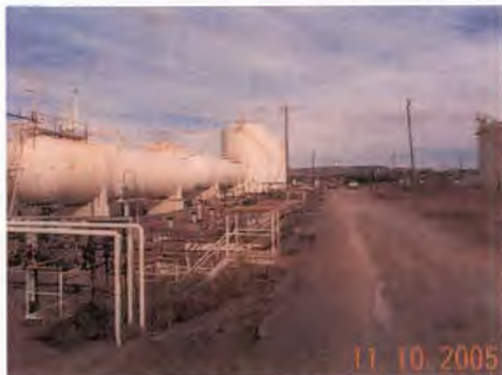
Looking W gas bullet tanks in background, which do not require berms- gas at STP
