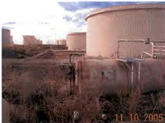
Looking S at tank batteries with constructed berms
