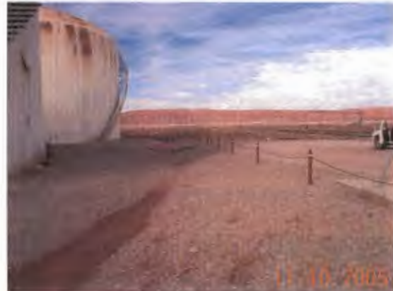
Close up of tanks without berms on the NE side of the facility looking N-NW
