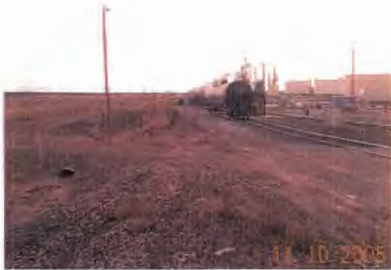
Railroad lagoon rack remediation area- NMED awaiting final remediation report
