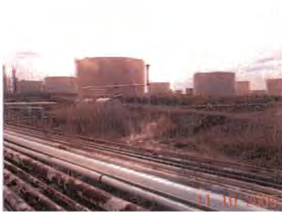
Pipe rack trending N-S on east side of facility
