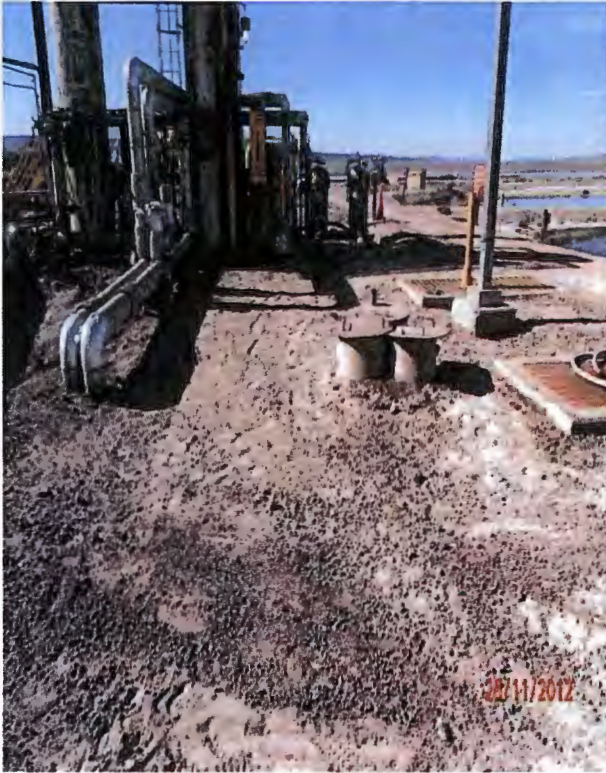
East side of the benzene strippers
